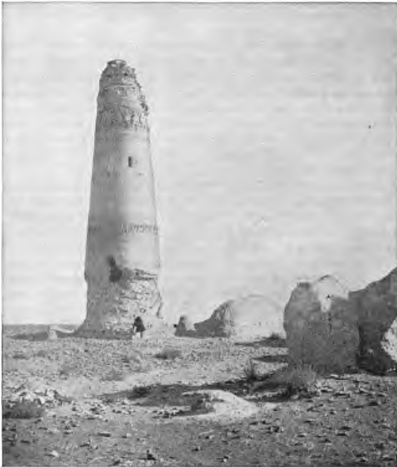
FIG. 118.—A Ruined Tower in Eastern Persia.
